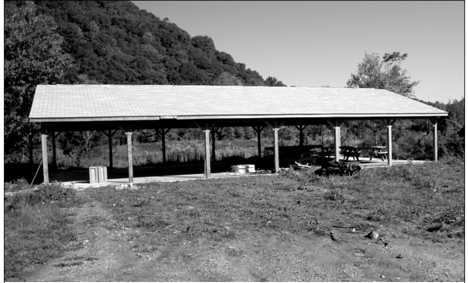
Newly completed AMD&ART Park recreational pavilion. With funding from the United States Forest Service, the pavilion was constructed by the Naval Mobile Construction Battalion 23.
